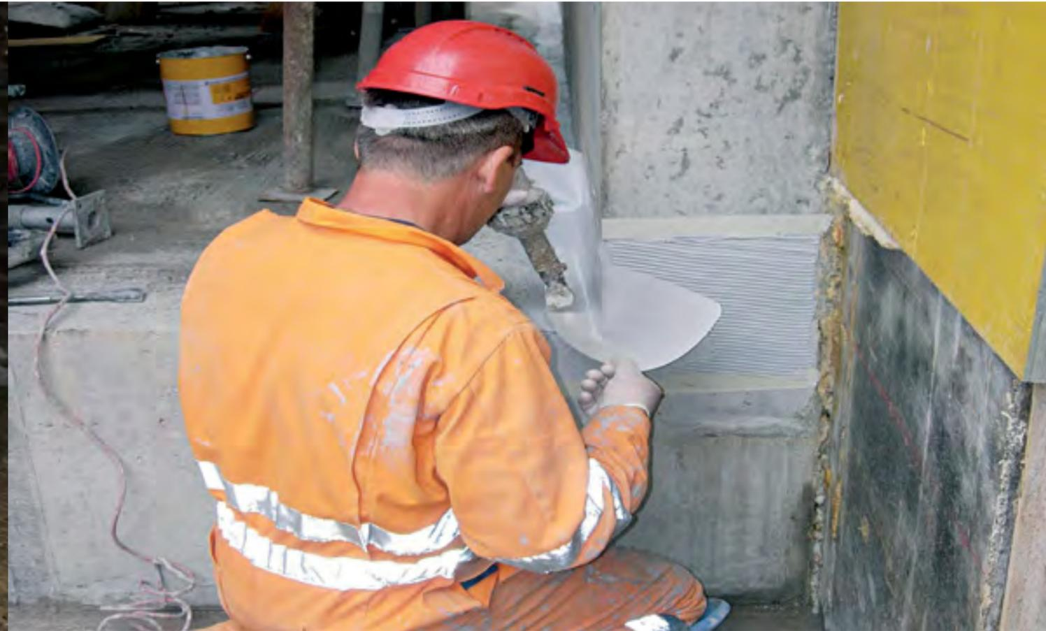
A high performance joint sealing system consisting of the Sikadur®-Combiflex® SG sealing strips and Sikadur® epoxy adhesive. This system is renowned worldwide for proven performance in sealing difficult joints and/or cracks in all types of watertight and retaining structures. It is particularly useful in watertight basement construction and can be applied both internally and externally to meet the specific project's requirements.
