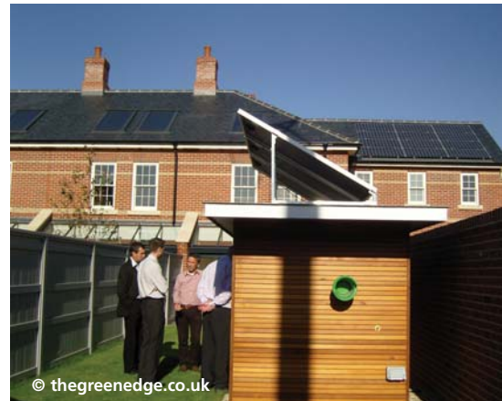
Figure 8: Energy Shed with ground source heat pump 600w array on roof and 3.4kW array on house
