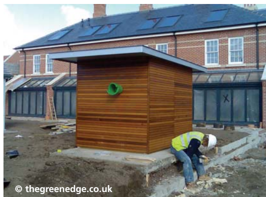
Figure 6: Energy Sheds being installed at Essex Energy Village
