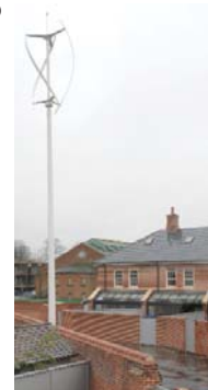
Figure 4: Vertical axis wind turbine with the Essex Energy Village
