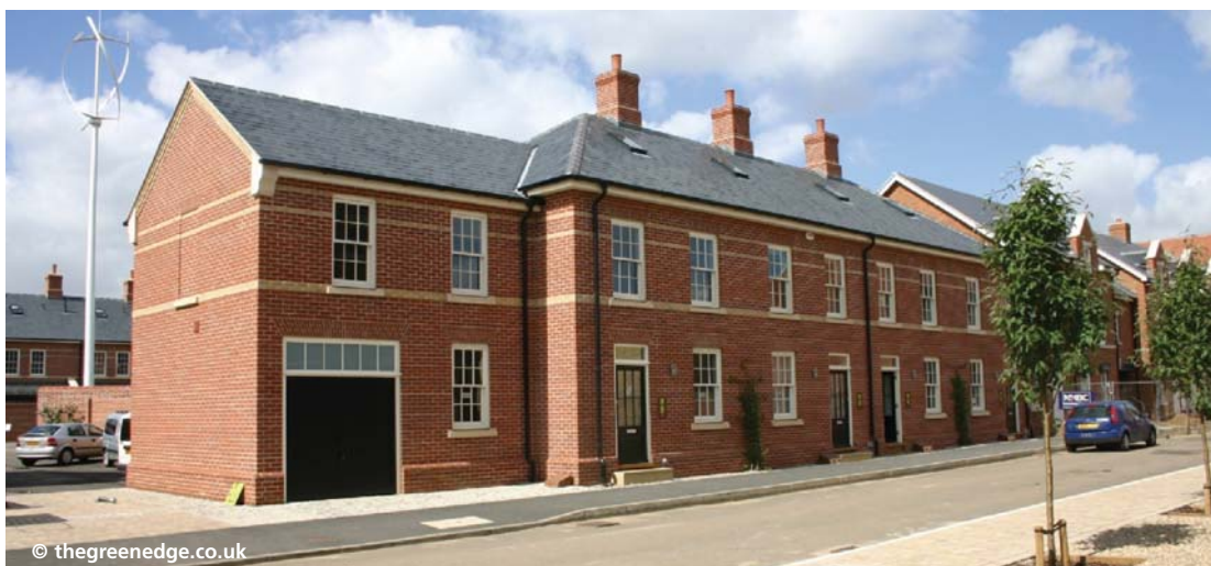
Figure 1: Four houses at the Essex Energy Village, north elevation
