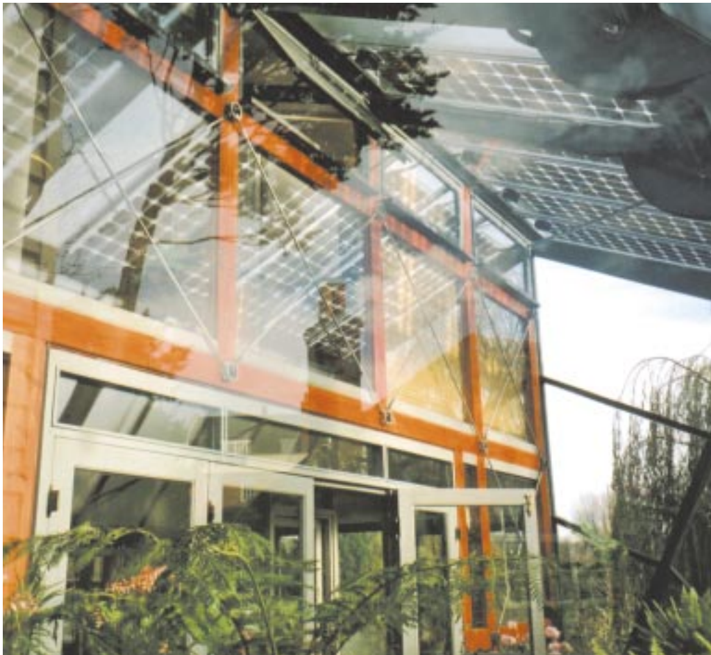
Hope House, interior view of conservatory
