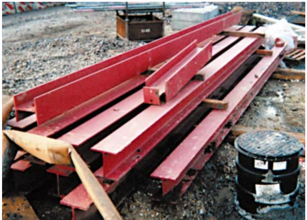
All the structural steel is reclaimed
